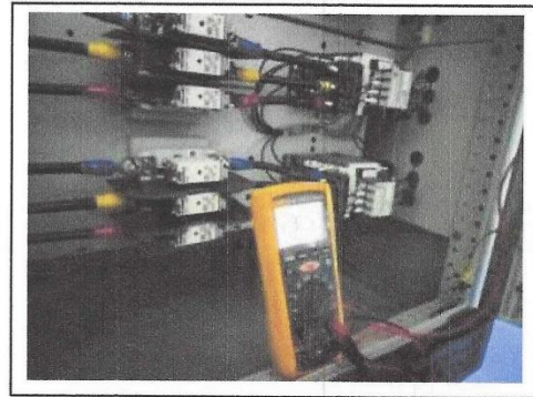
Picture 5 Capacitor bank preventive maintenance and Ground resistance test.
