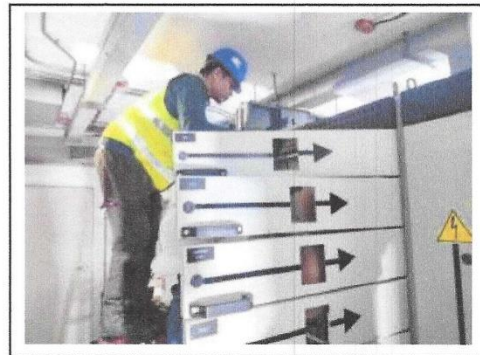
Picture 3 Main Distribution Board preventive maintenance.
