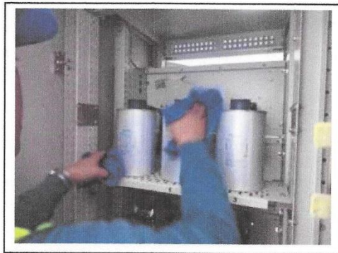
Picture 5 Capacitor bank preventive maintenance and Ground resistance test.
